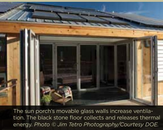
The sun porch's movable glass walls increase ventilation. The black stone floor collects and releases thermal energy. Photo © Jim Tetro Photography/Courtesy DOE.
