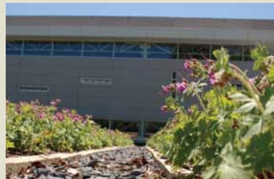
Bevan’s Variety Cranesbill Geraniums highlight the Anamosa limestone-edged blue stone runnels that direct excess surface water from garden areas to infiltration trenches that run through the King Pavilion site. *Photo by Alison Weidemann.*
