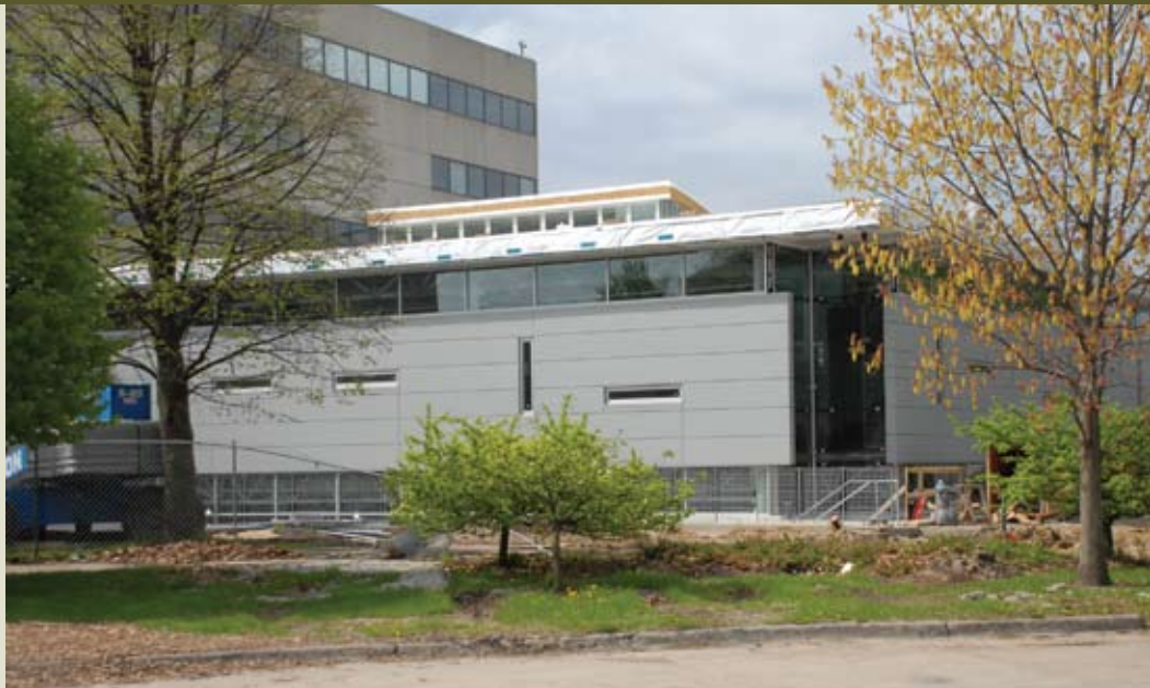
Construction was substantially completed on the King Pavilion in early May. As of press time, the building still awaits planting of its green roof, and crews continue to finish interior details. It will be open for fall classes and dedicated on August 24. Photo by Heather Sauer.
