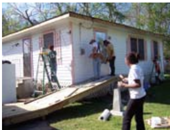
ADA ramp construction, post-Hurricane Katrina outreach studio, DSN S 446/546
